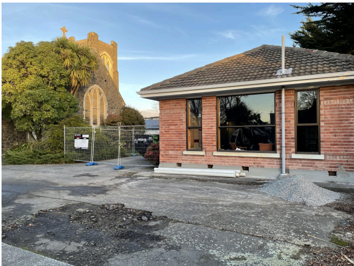
Strengthening work and improvements have begun.
